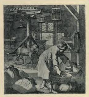
German in 1698, shews three spindles working three VII. pair of stones, all driven by the one blindfold horse. A curious mill drawn by two asses, shewn in a 16th century German engraving, appears to be more
