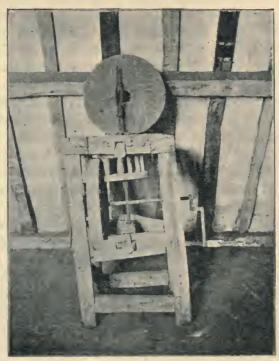
mounted on the spindle: which, passing through the lower stone, drives the upper. The latter, a Peak stone, is seen in the illustration reared upright in a position for shewing the grooving.
